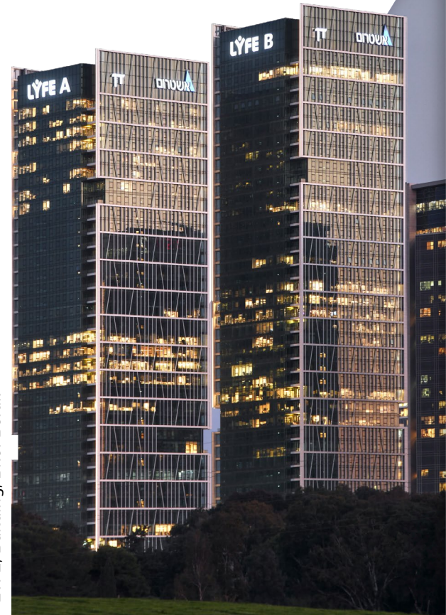
LYFE, Building, Bnei Berak
